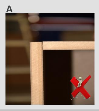
A.— Bad joints can appear by differences in panel thickness machining with drills "under table" systems.
